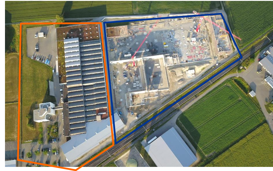
Land and buildings of MZ Infra in Sulgen
